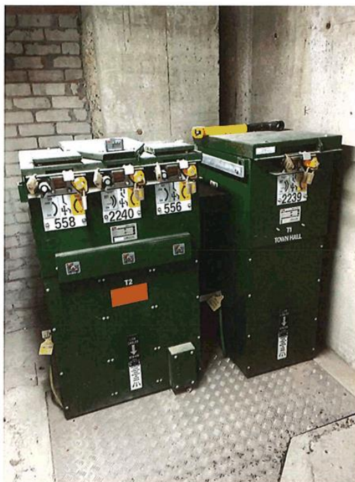
Transformers within room divided into two spaces
