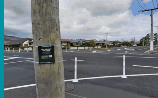
Kerb Build Outs – Argyle Street (Stage 1)
