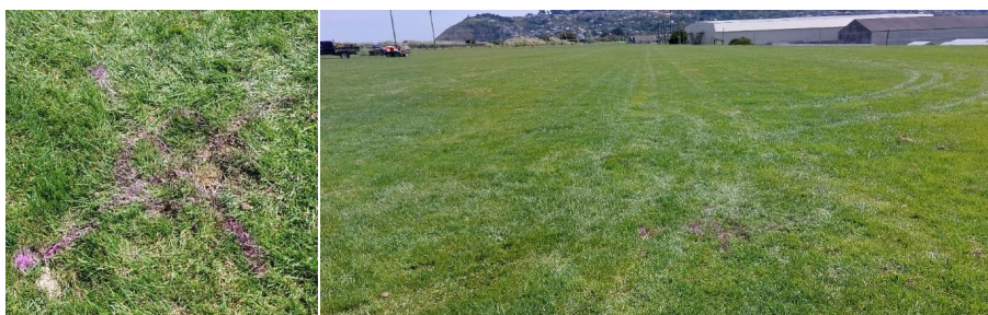
Photographs B17 (left) and B18 (right): example of reinstatement on completion of drilling, BH03 (taken 1.11.22).
