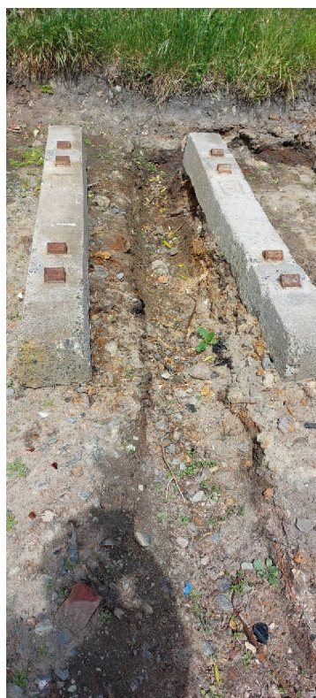
Photograph B6: Landfill materials such as brick, glass, concrete, timber, ash/charcoal daylighting among sleepers within the railway track at the northern boundary of Kettle Park (taken 3.11.22).
