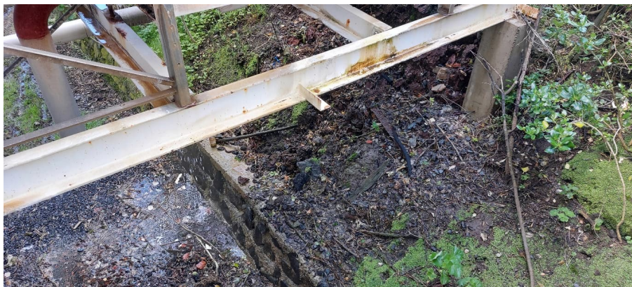
Photograph B5: Dunedin Ice Stadium cooling system overflow eroding bank materials below the railway track at the northern boundary of Kettle Park, landfill materials such as brick, glass, concrete, timber daylighting (taken 3.11.22).
