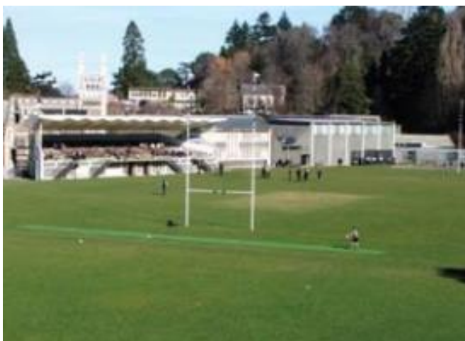
Figure 8: Littlebourne Ground and Grandstand
