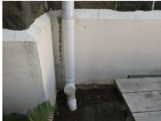
Photograph 19 – Showing the replacement uPVC rainwater downpipe and inspection point to the southern elevation.
