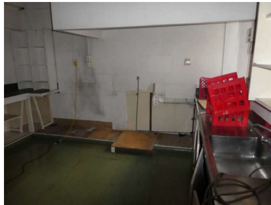
Photograph 216 – Showing the kitchen within the basement area.
