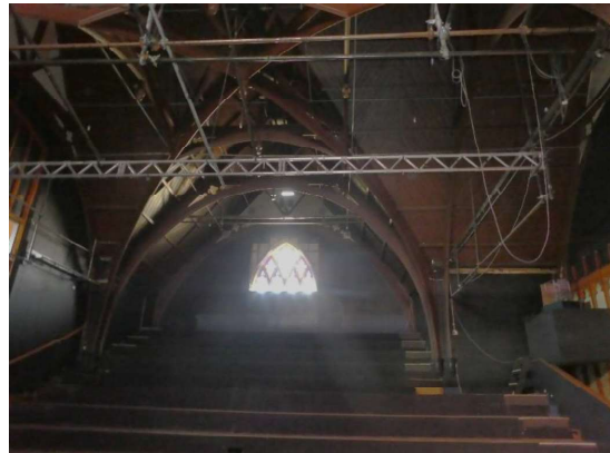
Photograph 83 – Showing the main theatre looking to the east.
