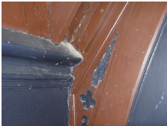
Photograph 120 - Showing typical painted timber rafter detail within the main theatre.
