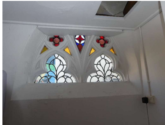
Photograph 173 – Showing the base of the leaded windows to the south western corner elevations from within the kitchen.
