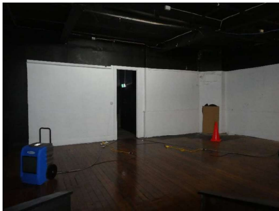
Photograph 100 - Showing the basement studio theatre space.
