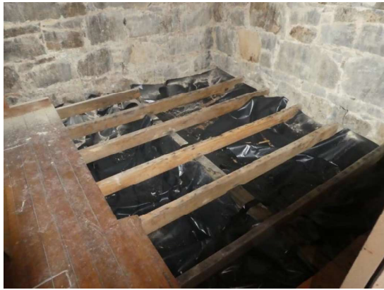
Photograph 143 - Showing the floorboards partially removed to the Dressing Room 2 behind the studio theatre within the basement.
