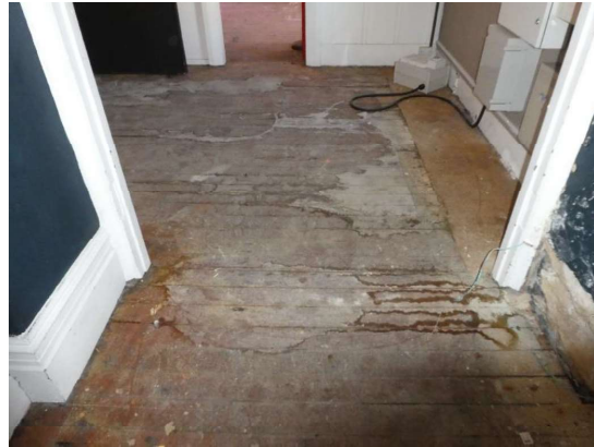
Photograph 134 – Showing the timber floor boards to the south eastern vestibule.
