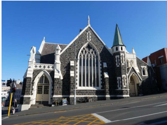
Photograph 24 - Showing the eastern elevation.
