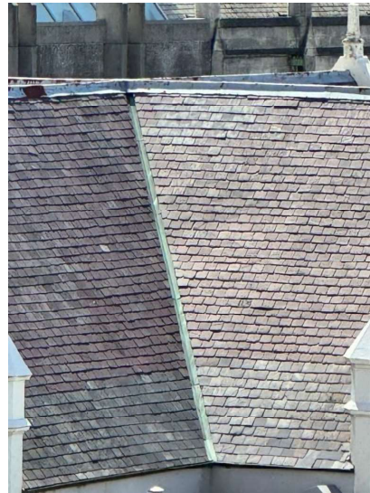
Photograph 2 – Showing the south western roofs and copper valley gutter.
