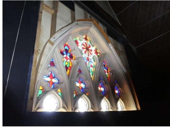
Photograph 183 – Showing the southern stained glass to the lancet tracery window on the southern elevation above the seating area of the theatre.
