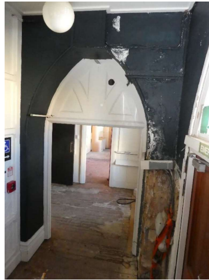
Photograph 93 – Showing the south eastern entrance and vestibule.
