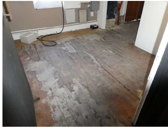
Photograph 136 – Showing the timber floor boards to the south eastern vestibule.
