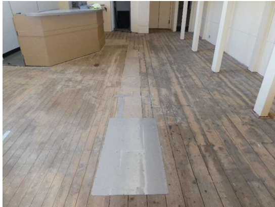
Photograph 133 - Showing the timber floor boards and target repairs within the bar area.
