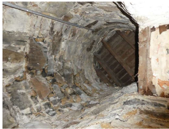
Photograph 161 – Showing the ceiling / timber floor installed within the bell tower looking up from the basement area.
