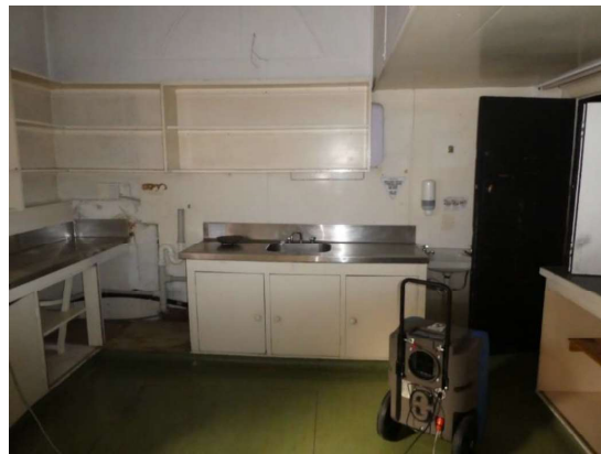
Photograph 218 – Showing the kitchen within the basement area.
