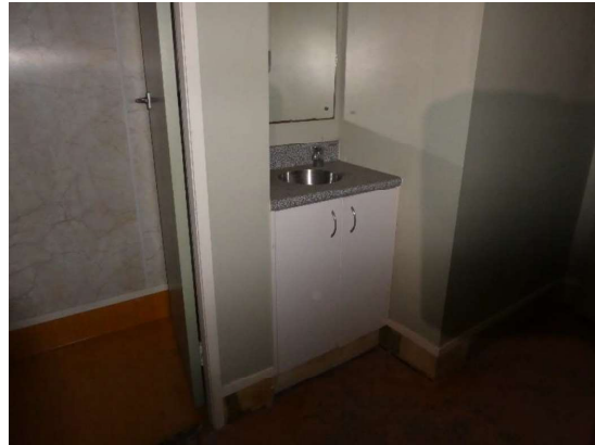
Photograph 225 – Showing the wash hand basin in the male toilet.
