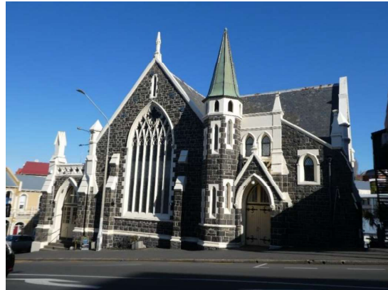
Photograph 25 – Showing the eastern elevation.
