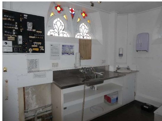
Photograph 81 – Showing the southern kitchen adjacent to the bar area. Noting electrical sub-distribution board to the southern wall.
