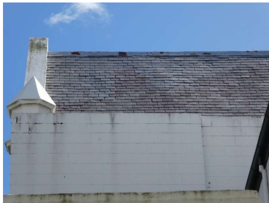
Photograph 3 – Showing the south western roofs and flat roof area above the extension.
