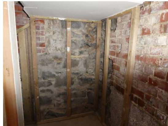
Photograph 200 – Showing the linings removed from the basement floor to the former project managers office at the north western stairwell.
