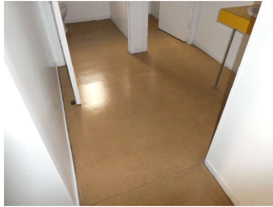
Photograph 140 – Showing the vinyl to the basement female toilets.
