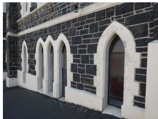
Photograph 57 – Showing the steel framed windows on the southern elevation.
