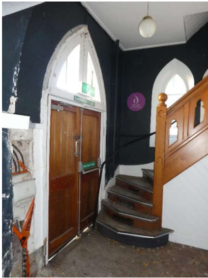
Photograph 92 - Showing the south eastern entrance and vestibule.
