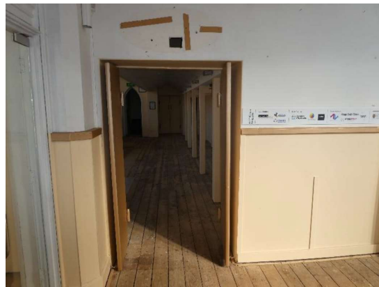
Photograph 76 – Showing the double doors leading from the entrance foyer to the bar.
