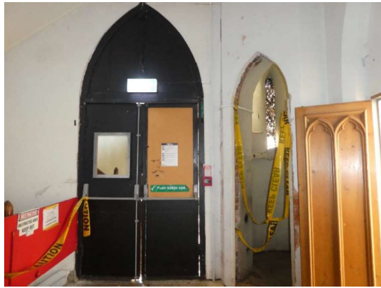
Photograph 188 - Showing the north western entrance door and the open internal panel door to the north western vestibule.
