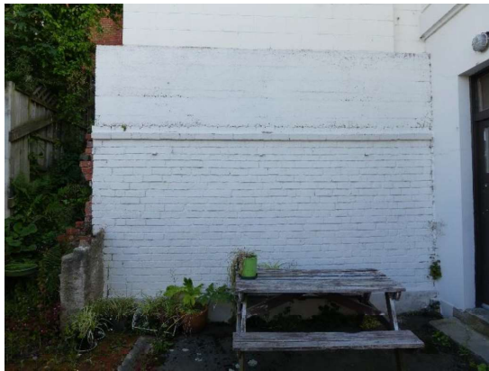
Photograph 41 – Showing the two-story extension to the south western corner.
