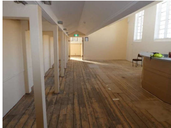
Photograph 80 – Showing the southern bar area looking towards the entrance foyer.
