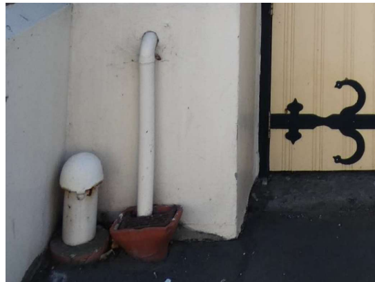
Photograph 265 – Showing the uPVC pipework to external clay gully adjacent to the southern entrance door .
