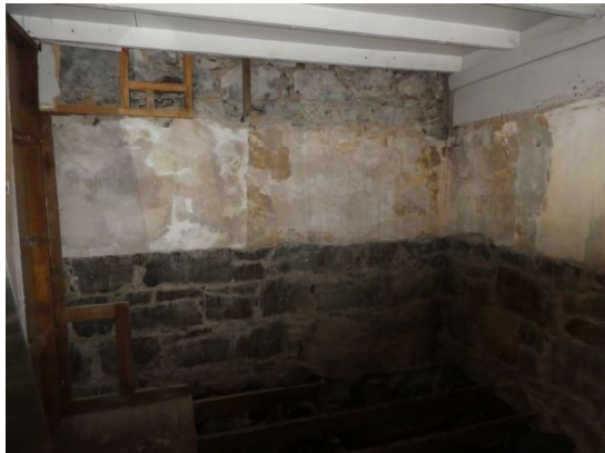
Photograph 108 - Showing the unlined / plastered walls to Dressing Room 2 accessed off the Green Room.
