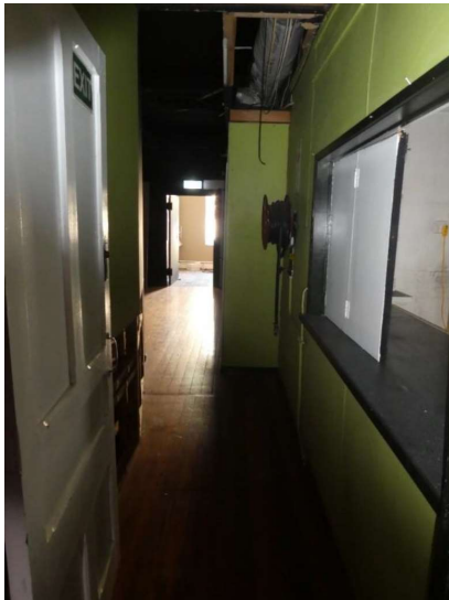
Photograph 112 - Showing the corridor formed behind the studio theatre seating.
