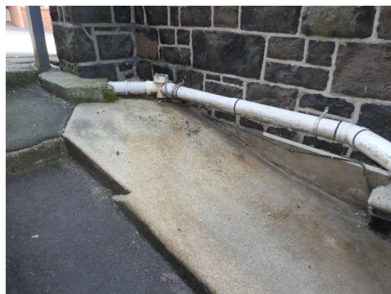
Photograph 21 – Showing the uPVC rainwater pipework to the western elevation.
