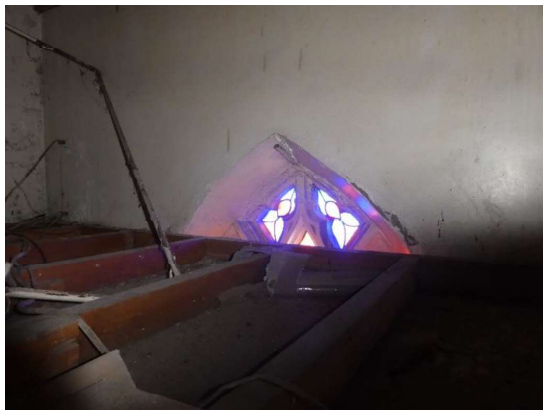
Photograph 67 - Showing the ceiling joists and the hidden top to the leaded lancet window within the roof space above the kitchen / bar.
