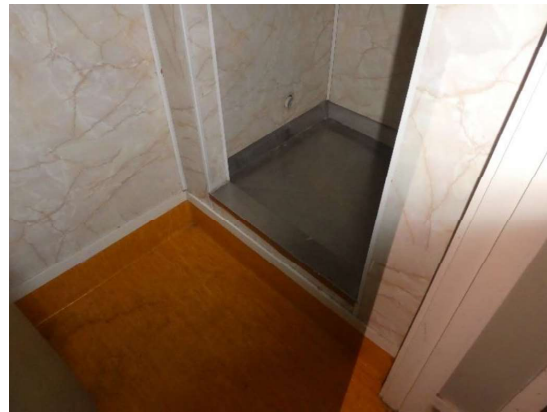
Photograph 223 – Showing the stainless steel shower tray and Seratone linings.
