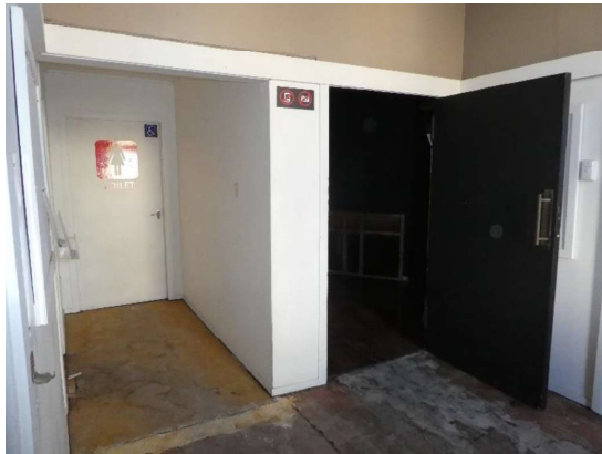
Photograph 94 - Showing the lobby to the toilets and basement theatre.
