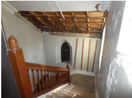
Photograph 116 - Showing the open underside of the roof structure to the north eastern stairwell.
