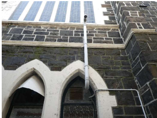
Photograph 54 - Showing the steel framed windows on the western elevation. Noting inappropriate positioning of services.
