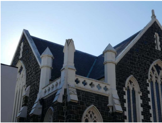
Photograph 7 - Showing the slate roof to the south eastern corner.
