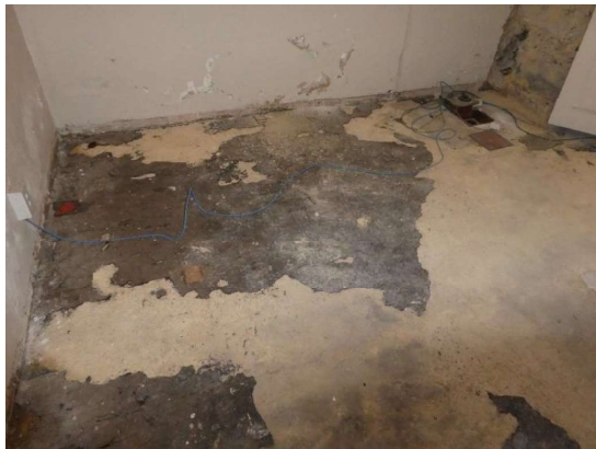
Photograph 137 - Showing the floor to the former basement administration office.
