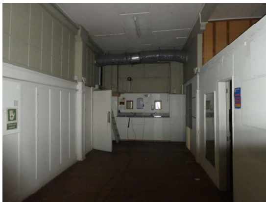
Photograph 102 - Showing the Green Room and kitchenette behind the basement studio theatre. The upper levels appear to be the original glazing which has been painted.
