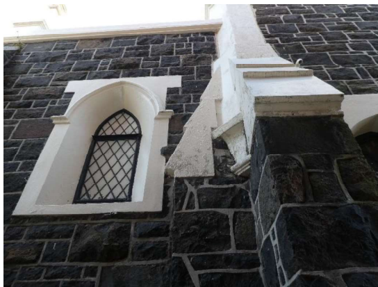
Photograph 60 - Showing the leadlight lancet window and buttress to the north eastern elevation.
