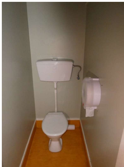
Photograph 226 – Showing the cubicle to the female toilet.
