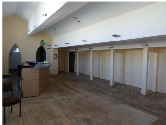
Photograph 78 – Showing the eastern bar area.
