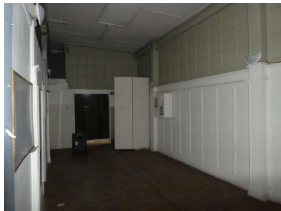
Photograph 103 – Showing the Green Room behind the basement studio theatre. The upper levels appear to be the original glazing which has been painted.
