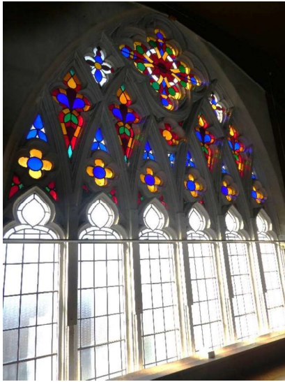
Photograph 166 - Showing the stained glass to the eastern tracery window within the meeting / theatre technical room.
