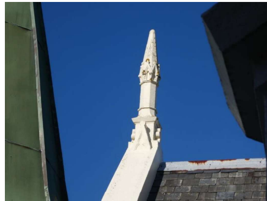
Photograph 27 - Showing the pinnacle to the northern gable.
