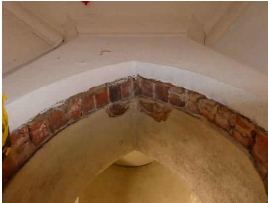
Photograph 158 - Showing the exposed brick arch to the bell tower.
