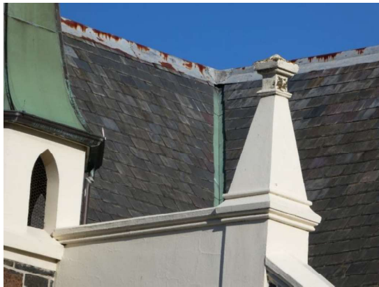
Photograph 26 - Showing typical pinnacle detail to the northern elevation.
