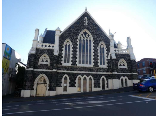
Photograph 23 – Showing the southern elevation.
