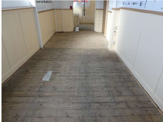
Photograph 131 - Showing the timber floor boards to the main entrance foyer.
