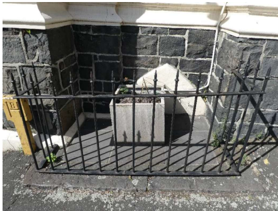
Photograph 237 - Showing the iron railings and blocked up basement windows to the north elevation.
