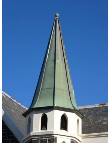
Photograph 15 – Showing the replacement copper roof to the bell tower.
