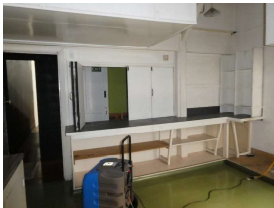
Photograph 217 - Showing the kitchen within the basement area.
