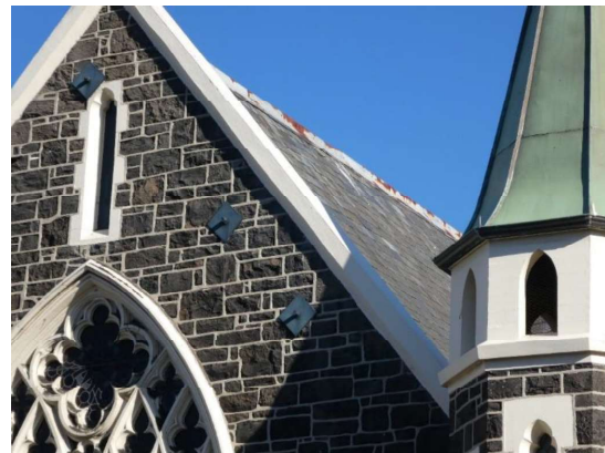
Photograph 30 – Showing the metal tie rods to the northern gable.
