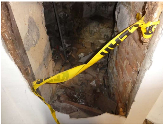
Photograph 160 - Showing the bell tower / turret from within the basement area.
