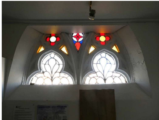
Photograph 172 - Showing the base of the leaded windows to the south western corner elevations from within the kitchen.
