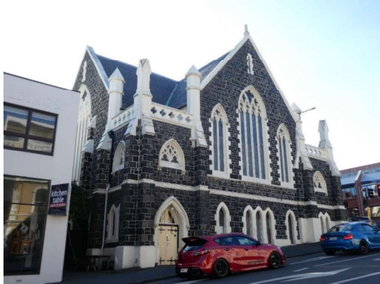
Photograph 22 - Showing the south western elevations.
