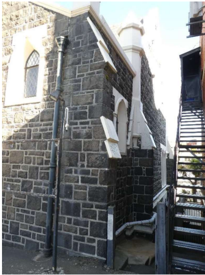
Photograph 17 - Showing the rainwater hopper and iron downpipe to the north western corner.
