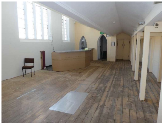
Photograph 77 - Showing the eastern bar area.
