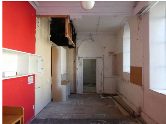
Photograph 97 – Showing the basement offices.
