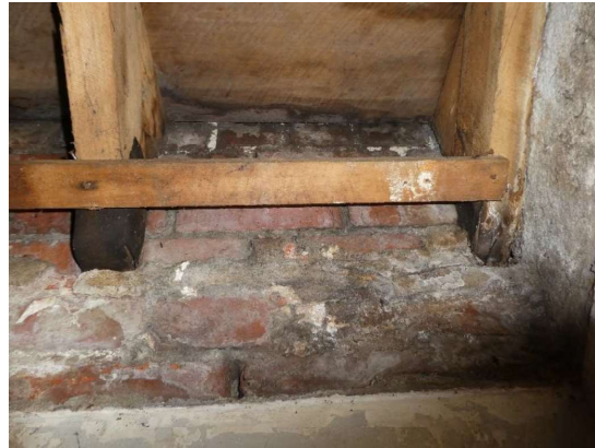
Photograph 119 – Showing the timber rafters built into the solid brick external walls to the western wall of the north western stairwell.
