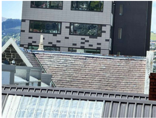
Photograph 1 – Showing the south western roofs and flat roof area above the extension.
