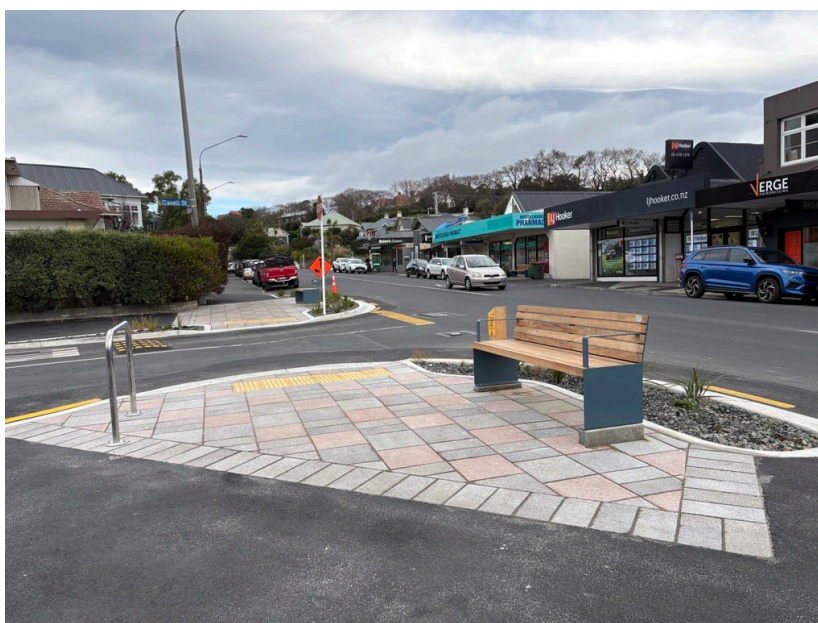
Looking east from the corner of Musselburgh Rise and Cavell Street – After
